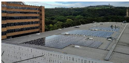
Despite the challenge to complete works during the COVID shutdowns, Estates & Facilities took the opportunity to undertake construction and improvement works including installing 422 Solar Photovoltaic panels on Technology Building which will generate 150,000 kWh of electricity annually.
